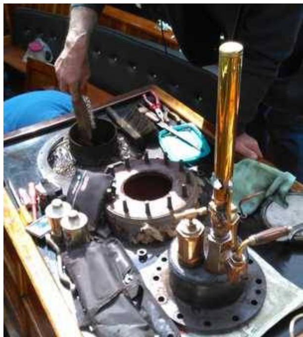
Figure C-4: Cleaning the Uptake
