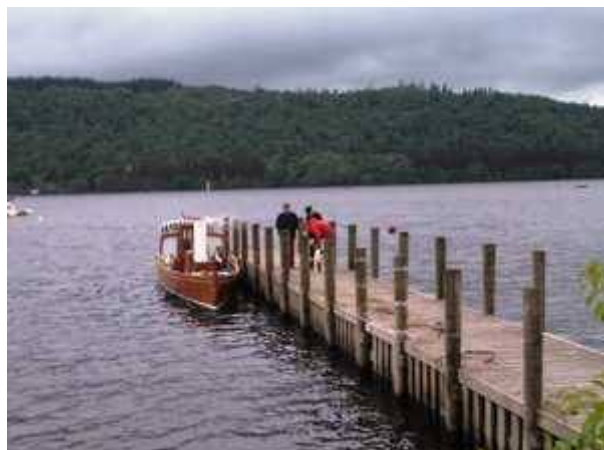
Figure 5-2: This Jetty may not need Fenders
